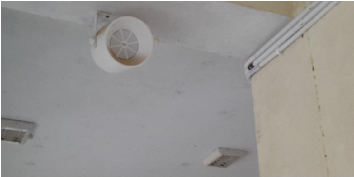
Photograph 39 Expansion of Infrastructure
